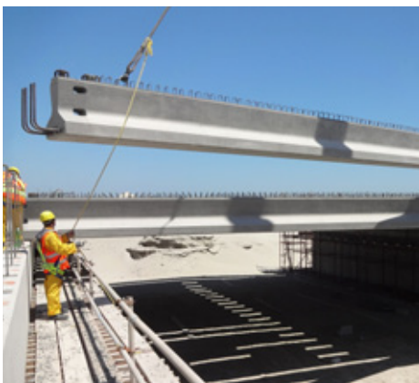
Distributor bridge construction, placing pre-cast beams
