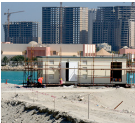
Electrical substation, scaffolding placed for external plastering and painting
