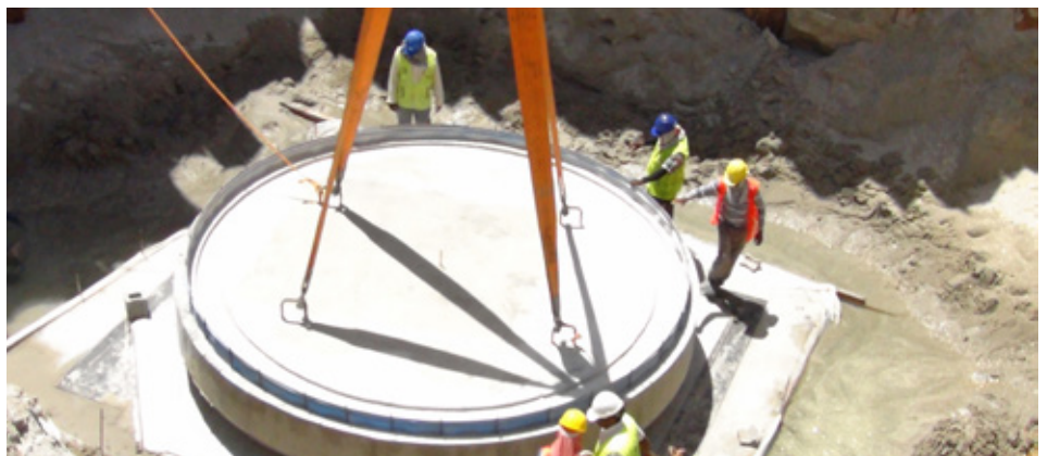
Placing first wetwell precast ring for a pumping station
