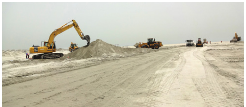
Road works, filling and land leveling works
